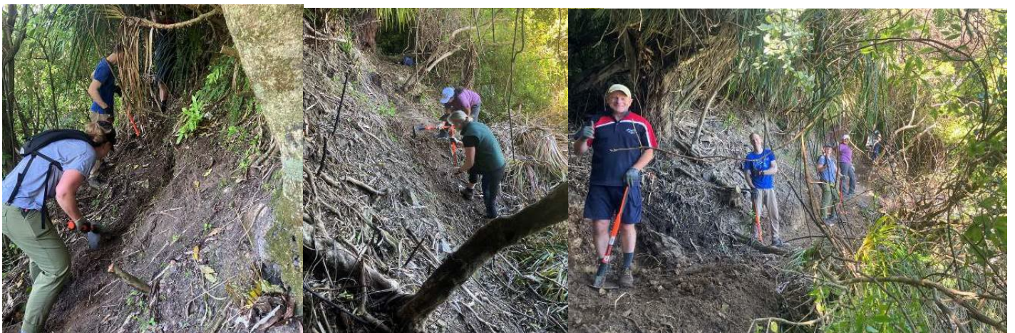
Benching out the new by-pass track
